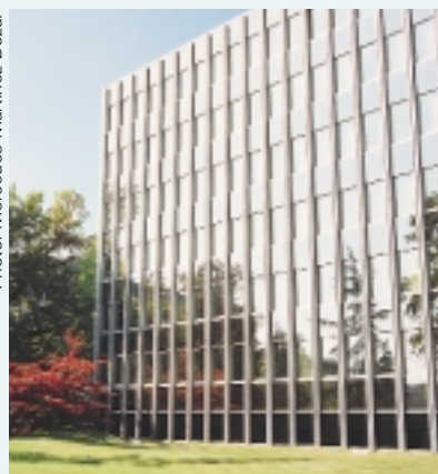
The Georg Bodenhausen Building, chemin des Colombettes, Geneva, designed by Pierre Brillard and constructed between 1958 and 1960, enlarged and modernized between 1988-89. It has six floors, one of which is underground.
