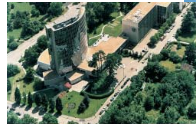
The new building will be linked to the Arpad Bogsch building and will provide 560 working places and 280 underground parking places
