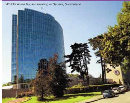
WIPO's Arpad Bogasch Building in Geneva, Switzerland.
