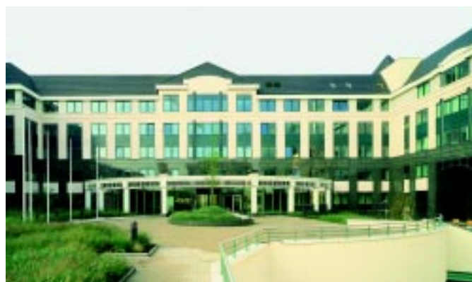
WCO headquarters in Brussels
