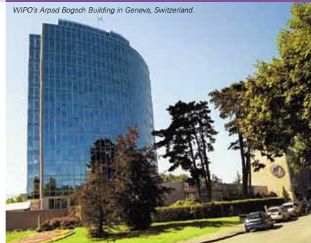
WIPO's Arpad Bogasch Building in Geneva, Switzerland.
