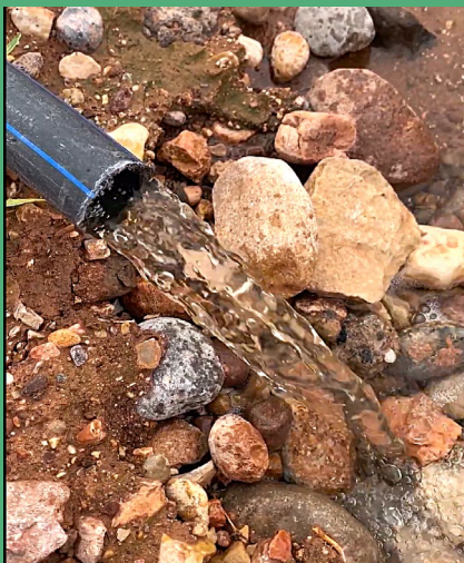
Treated water meets water quality standards
